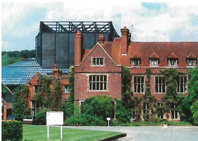
June 94: The new £33million Glyndebourne Opera House opened with a massive battery of sound, lighting and staging equipment.
