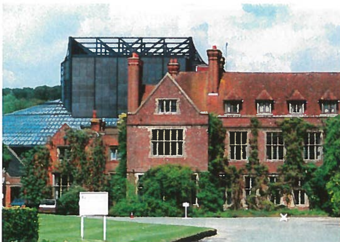
June 94: The new £33million Glyndebourne Opera House opened with a massive battery of sound, lighting and staging equipment.
